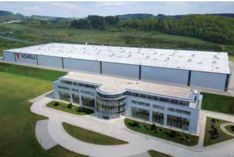
Plant 1 Production with administration and training centre
