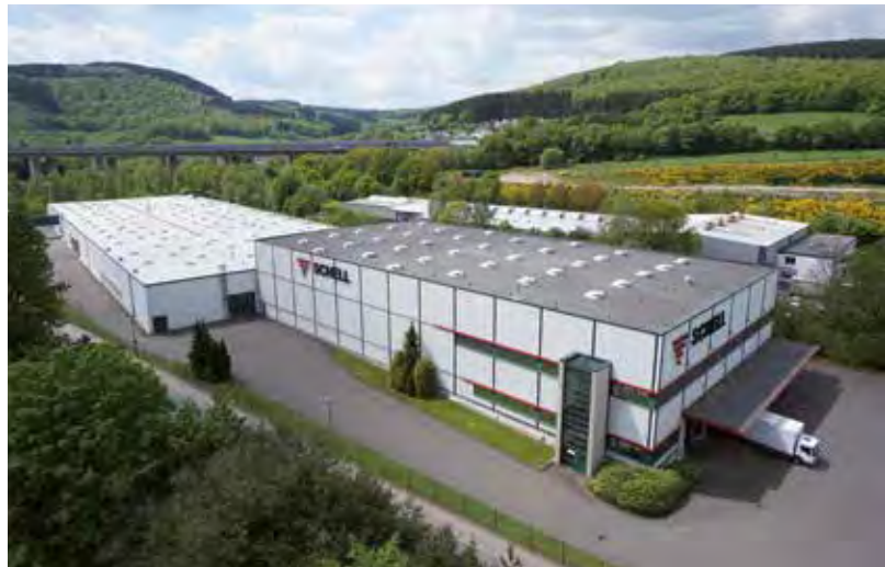
Plant 2 Production with logistics centre
